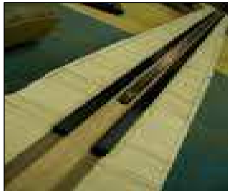
Fig 5: Fixing of Carbon rods over the beams as negative reinforcements
