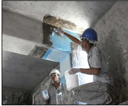
Fig 7: Saturation of surface with epoxy matrix
