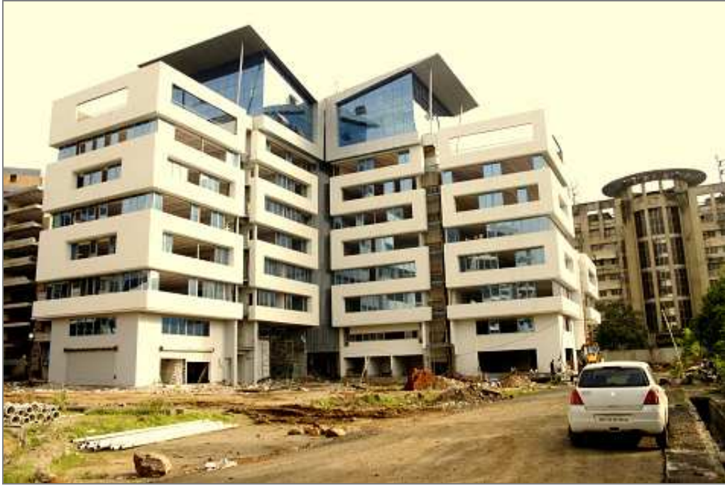
Fig 12: Final Building of the D-Block of the commercial complex after completion of all works.
