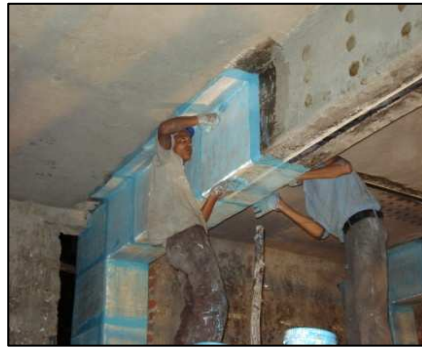
Fig 8: Fiber application and roller application.
