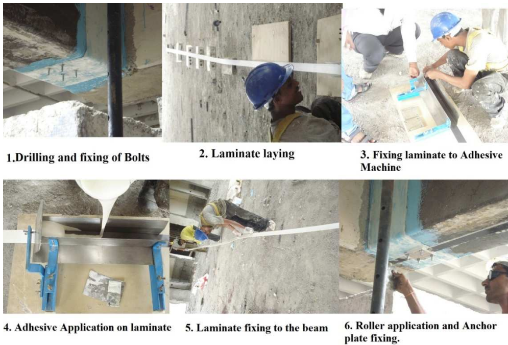
Fig 6: Fixing of laminate below the beams for flexural enhancement
