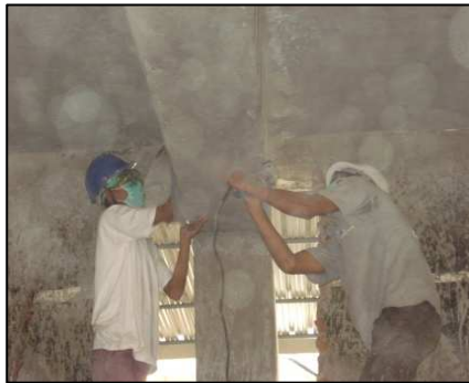
Fig 2: Surface preparation of beams
