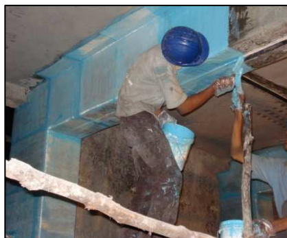
Fig 9: Application of second Coat of Epoxy matrix.
