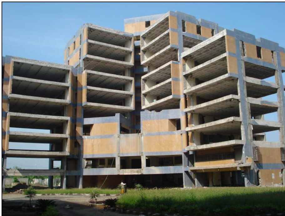
Fig.1 D-block of SEZ Commercial complex
