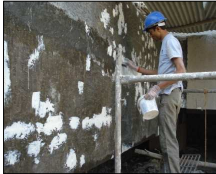
Fig 4: Filling uneven surface with leveling mortar
