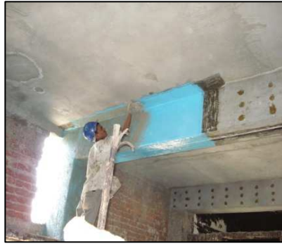
Fig 10: Sand Sprinkling for making surface rough for plastering and other finishing.
