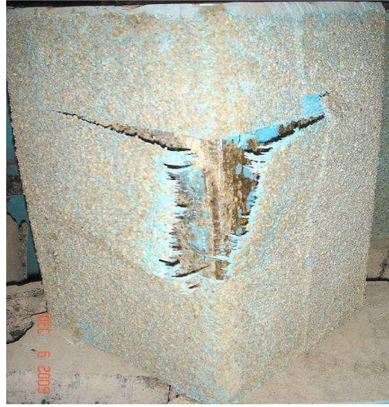
Fig 15 GFRP wrapped square prism with sharp edges 130 x 200 mm in size failure of fibers at corners due to stress concentration
