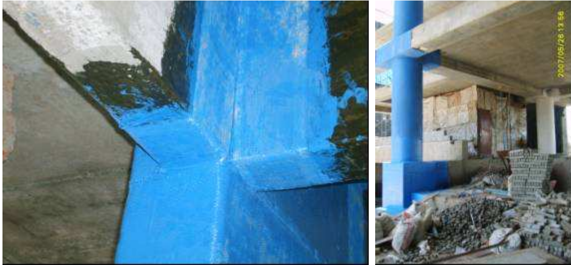
RC Columns after Completion of FRP Wrapping
