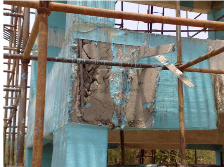
Fig 6 Failure of Beams of as built and retrofitted structure
