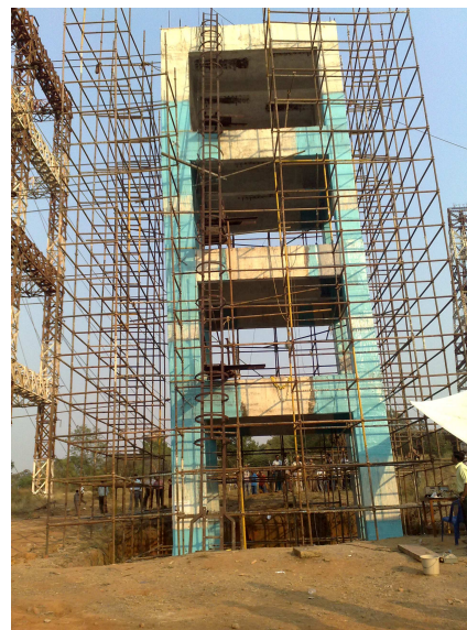
Fig 2 Testing of Retrofitted Structure
